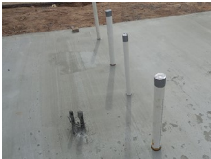
Plumbing students hit their marks and are inside the plumbing wall as they should be
