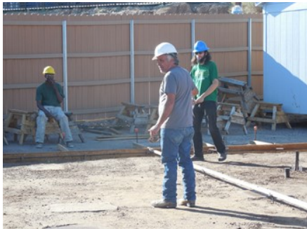
Carpentry Instructor Joseph Hirschfield oversees the project the morning of the concrete pour
