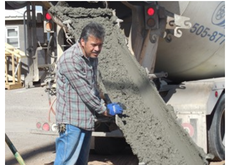
Doug Toca guides and controls the flow of concrete allowing instructors and students to concentrate on the task at hand.
