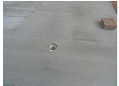
Pipes are removable with a simple pull to allow versatility in wall framing
