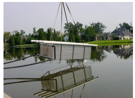
Installation in a n existing pond Image Credit: AWEB Supply ( http://www.awebgeo.com/illustrarions.html )
