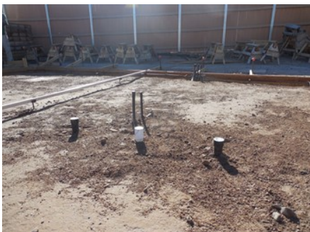
Plumbing students stubbed up pipe and topped with couplings and bushings set to finished grade
