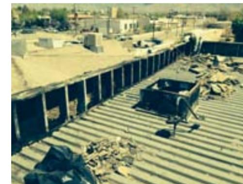
Severe roof damage due to fire.
