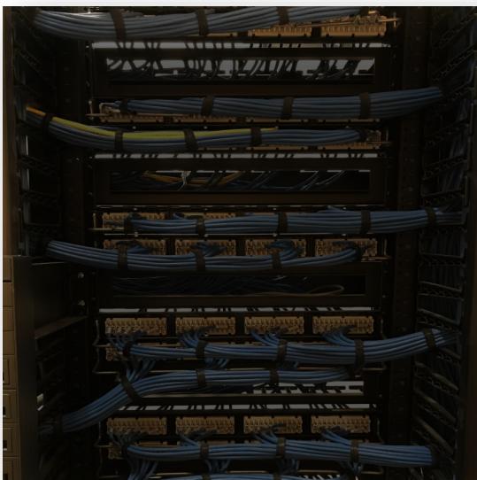
Building Cable Plant Installation
