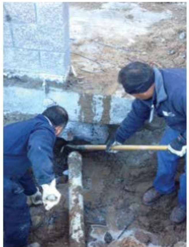
Crew works on plumbing problem at Tony Hillerman Middle School
