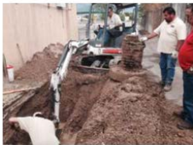
Many large repairs require the aid of heavy equipment.
