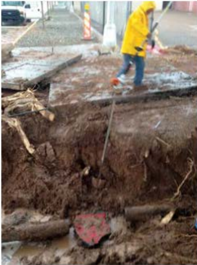
Plumbing jobs are often more than routine maintenance.
