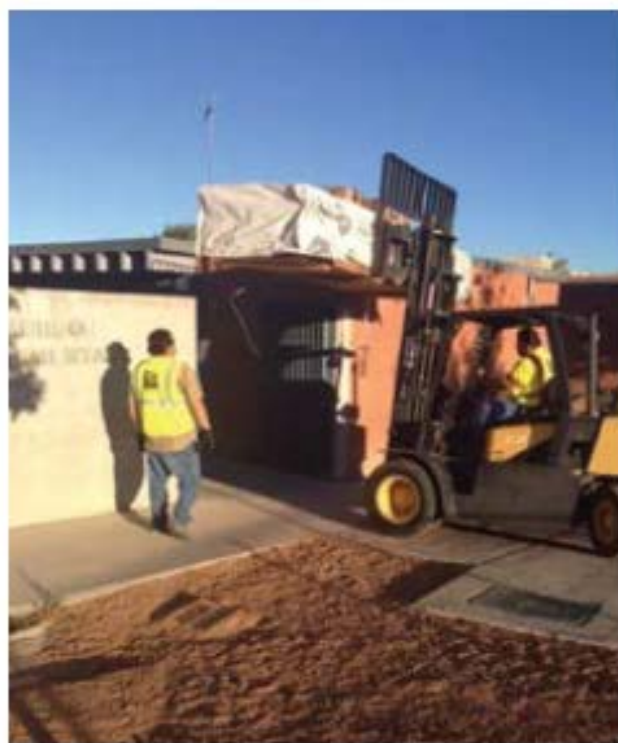
Delivering a pallet of garden supplies required lifting over the wall at Emerson Elementary School.
