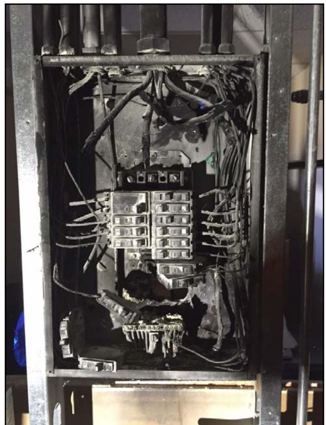
Electrical panel failure
