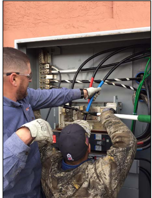
Installation of new electrical cabling
