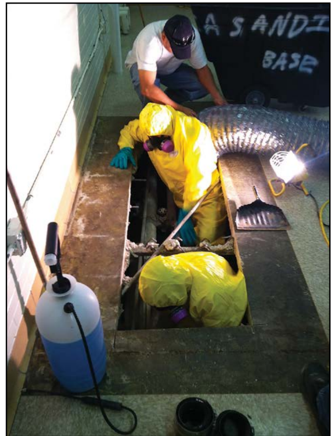
Asbestos abatement in tunnels below floor
