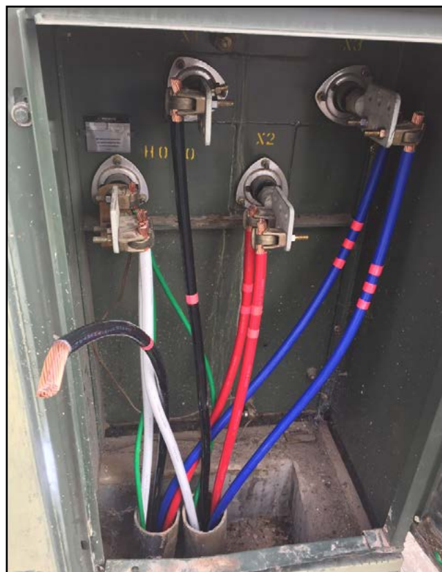
Electrical secondary upgrade
