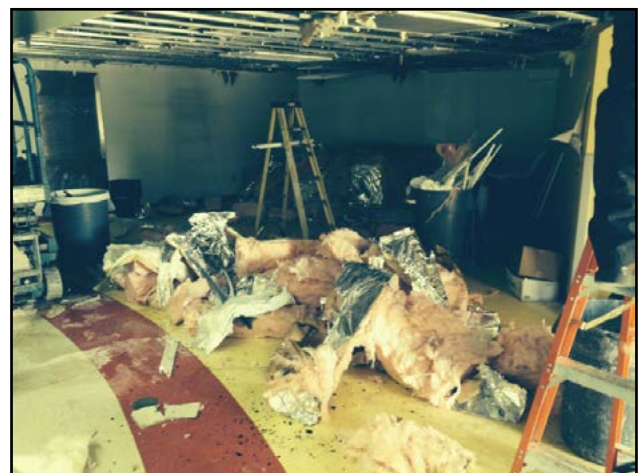
Major water line failure in school cafeteria causes severe damage
