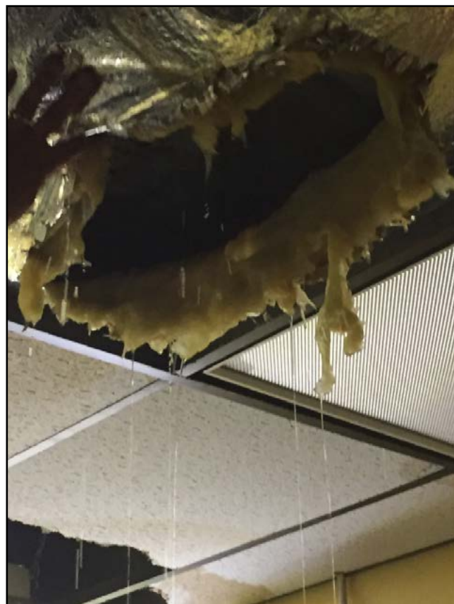
Water line break damage can be severe and require the services of several M&O departments
