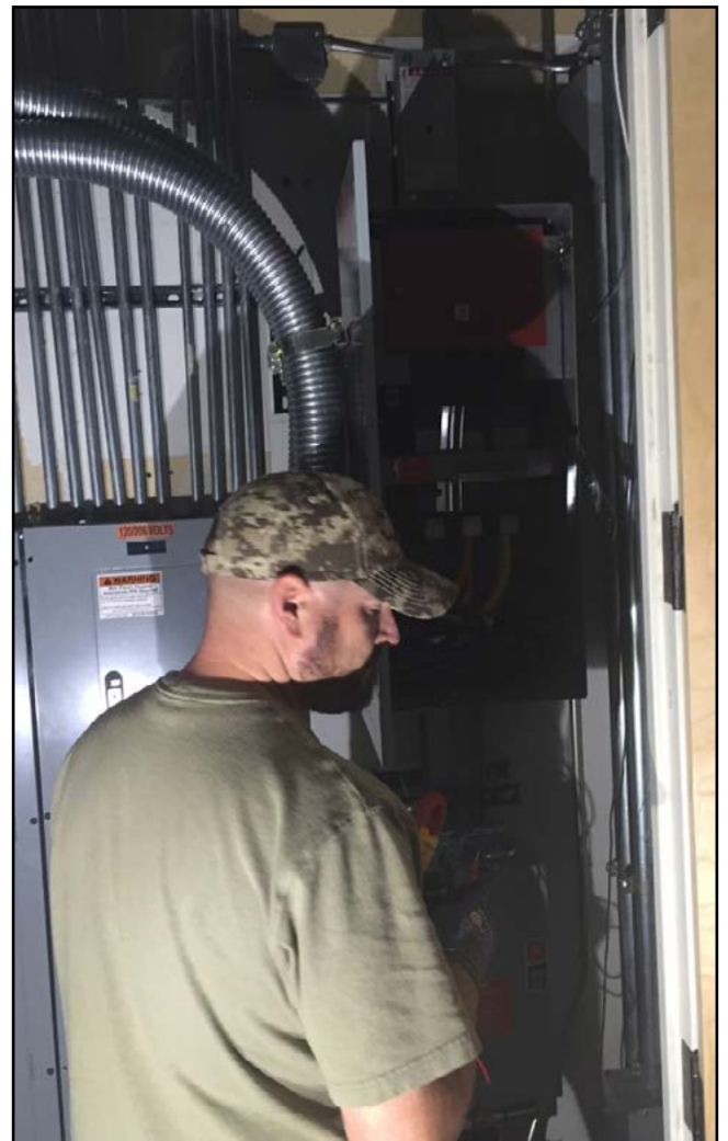
Tech working on an electrical upgrade
