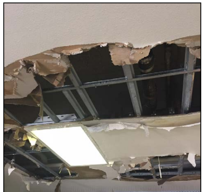
Ceiling damage due to broken water line
