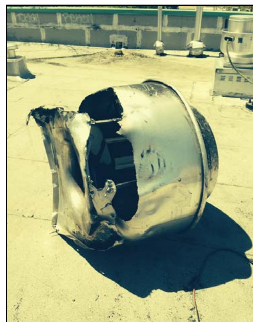
Mechanical equipment vandalism on high school roof
