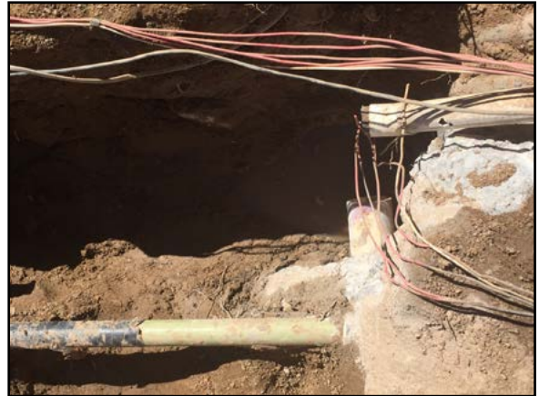
Damaged underground irrigation system
