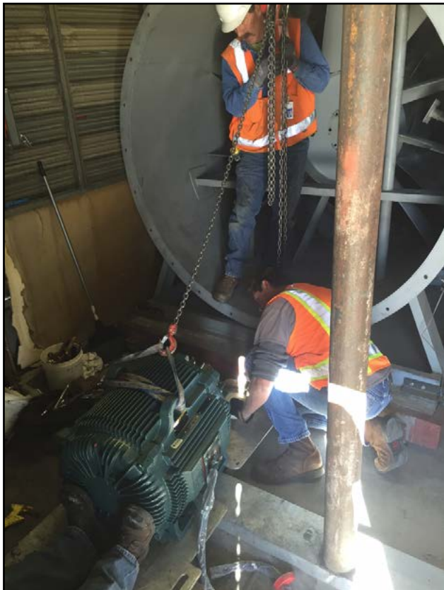
Motor replacement at City Center
