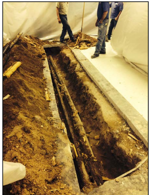
Replacement of old in-floor heating pipes at Hayes Middle School
