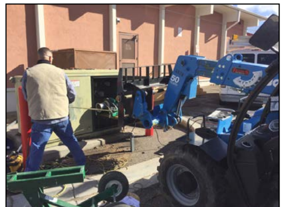
Replacing secondary electrical distribution system at Monte Vista Elementary School
