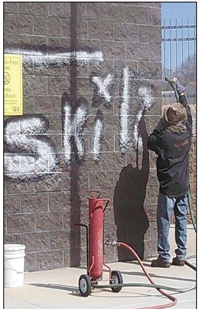
Graffiti sandblasting cleanup is never ending
