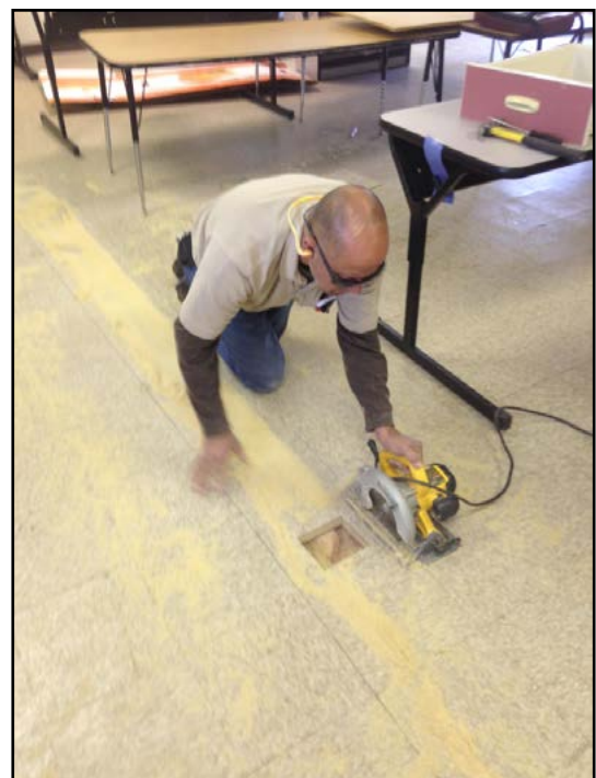
Floor repair in portable classroom.
