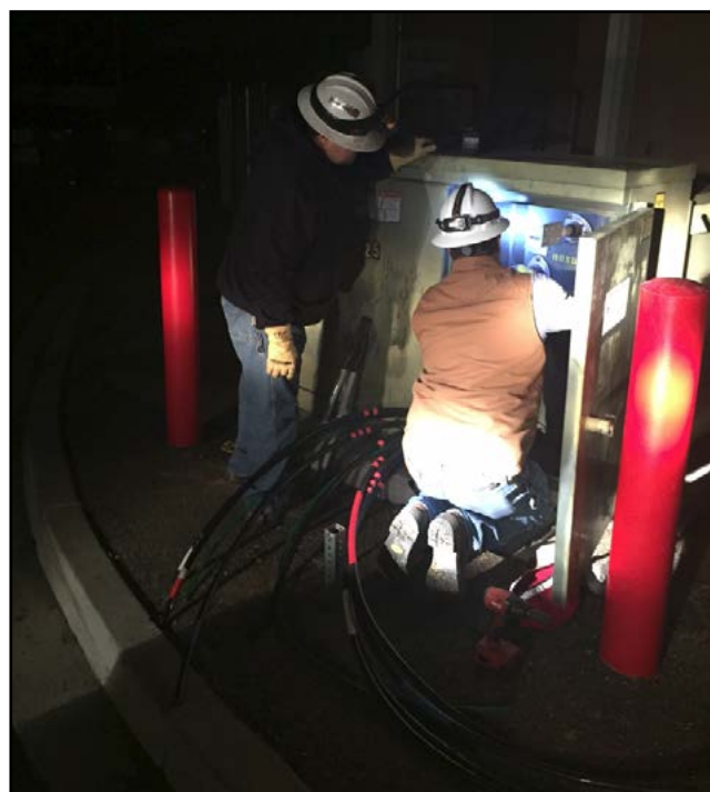
Emergency electrical repairs
