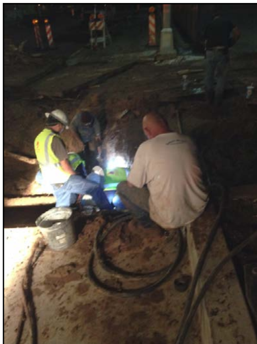
Emergency water line repair at Highland High School crews worked night and day
