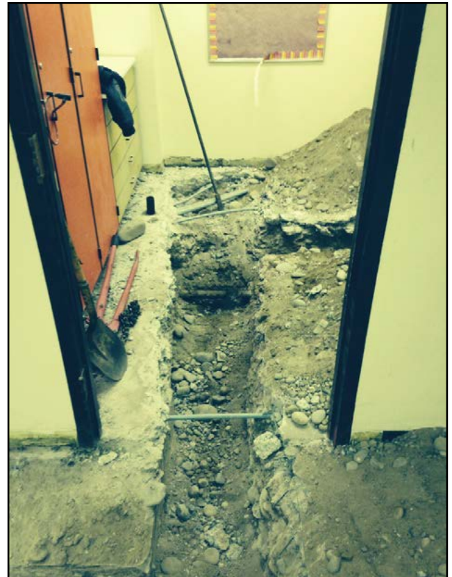
New plumbing installation in classroom
