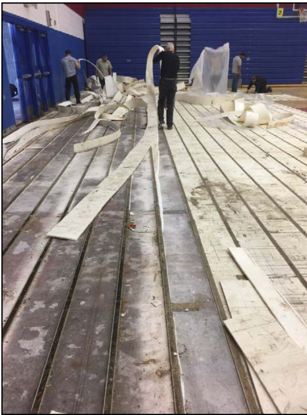
Installation of new flooring at West Mesa High School gym
